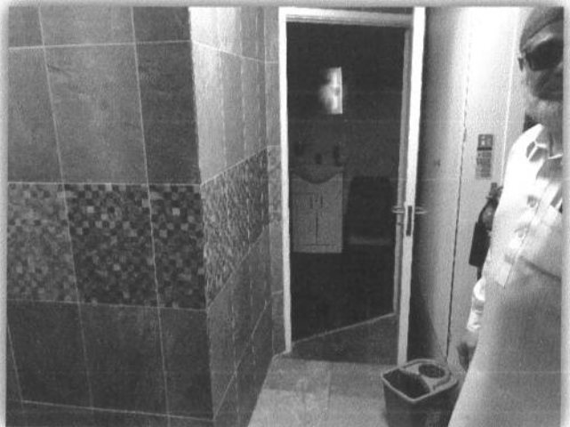
Image of the accessible toilet.
