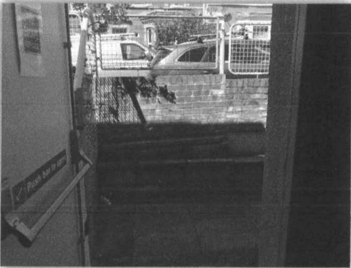
Image of the area for a potential platform lift.
