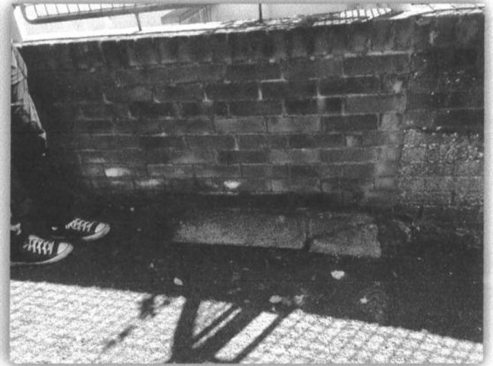
Image of the area for a potential platform lift.
