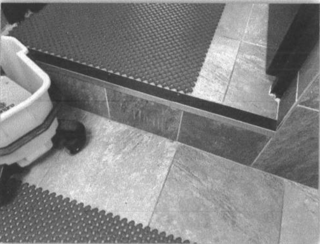
Image of the step down to the accessible toilet.
